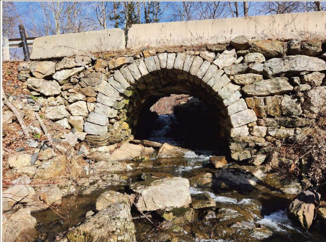
Photo No. 1: Downstream Elevation (Looking North)
